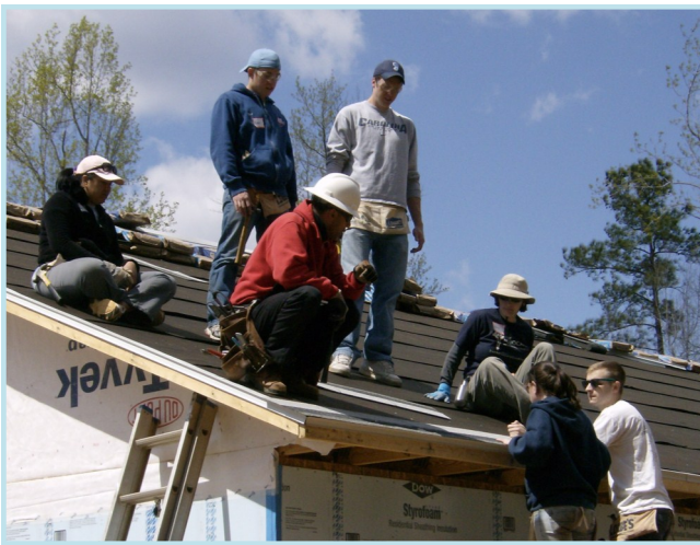
SHAC Habitat volunteers building a house in Northern Orange County
