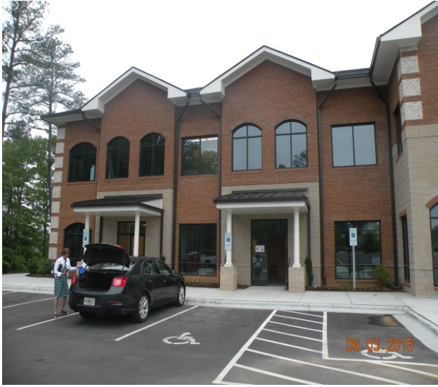
Front of building
