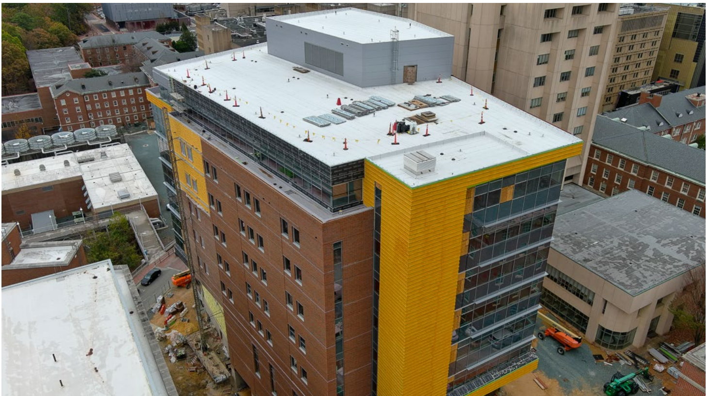
DRONE OVERVIEW – NORTH ELEVATION
