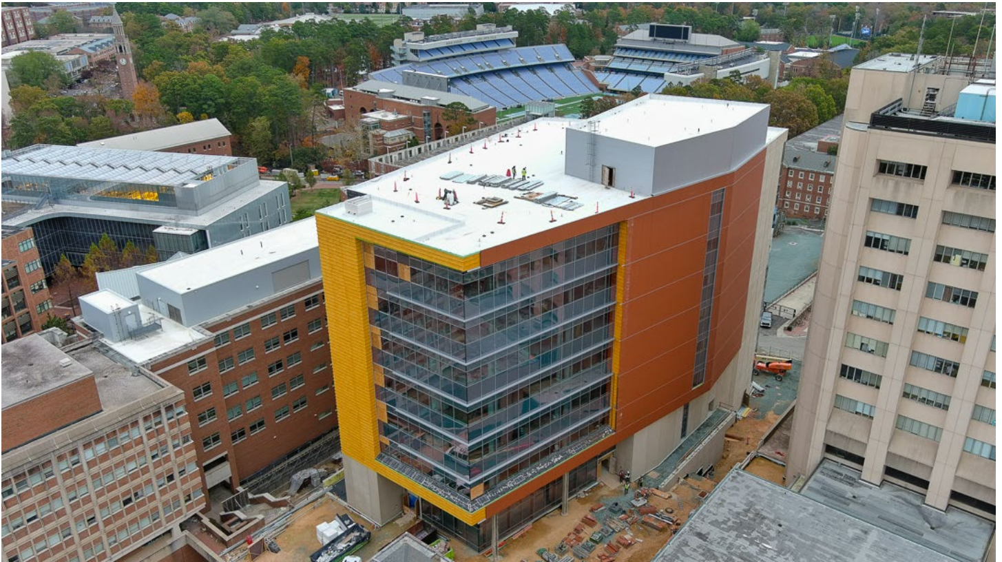
DRONE OVERVIEW – NORTH ELEVATION
