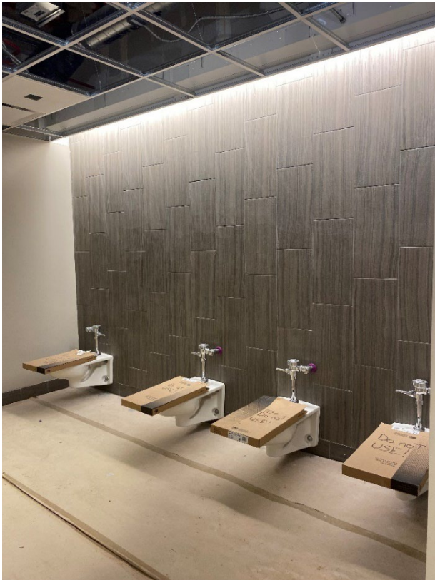
(2C) Level 4 Women's Bathroom (Above)
