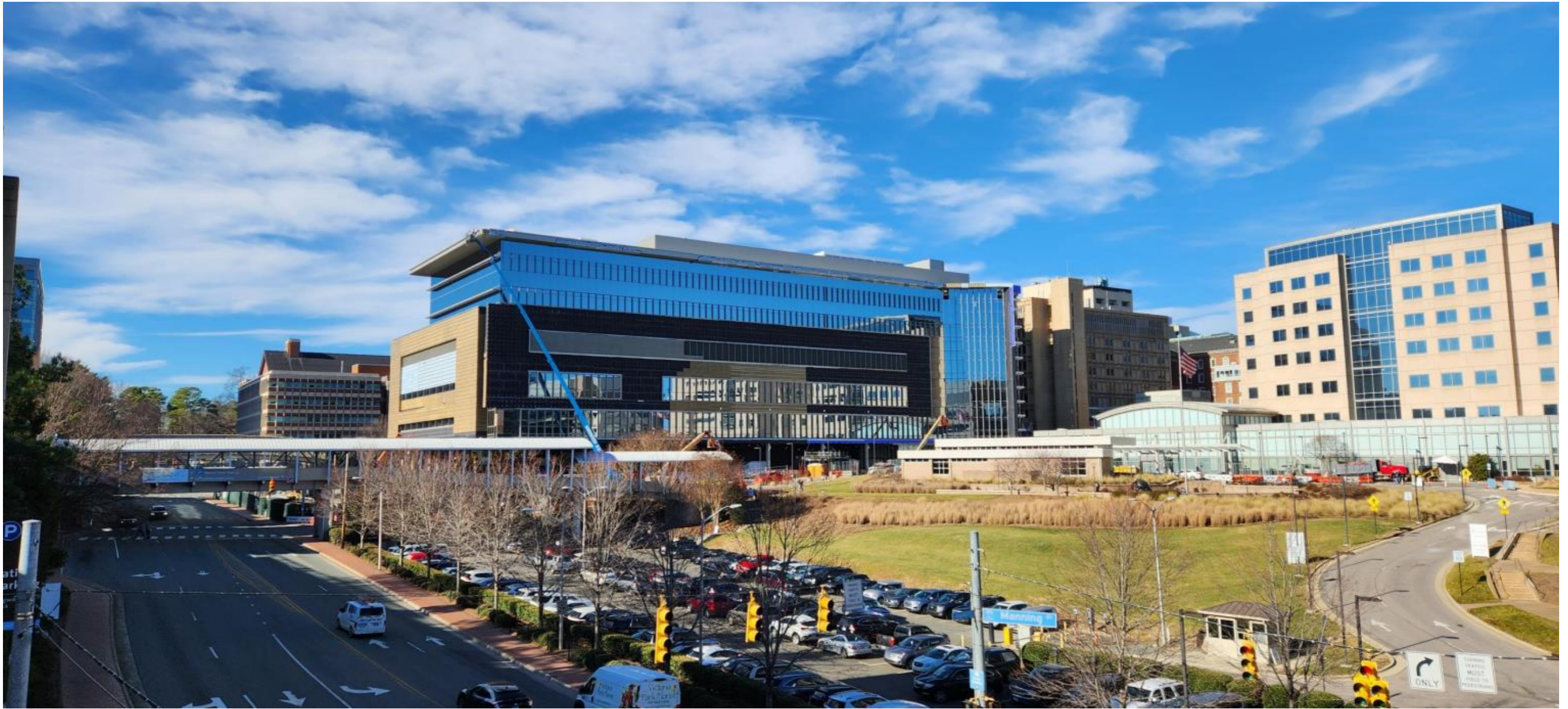
East Elevation – From Bridge C
